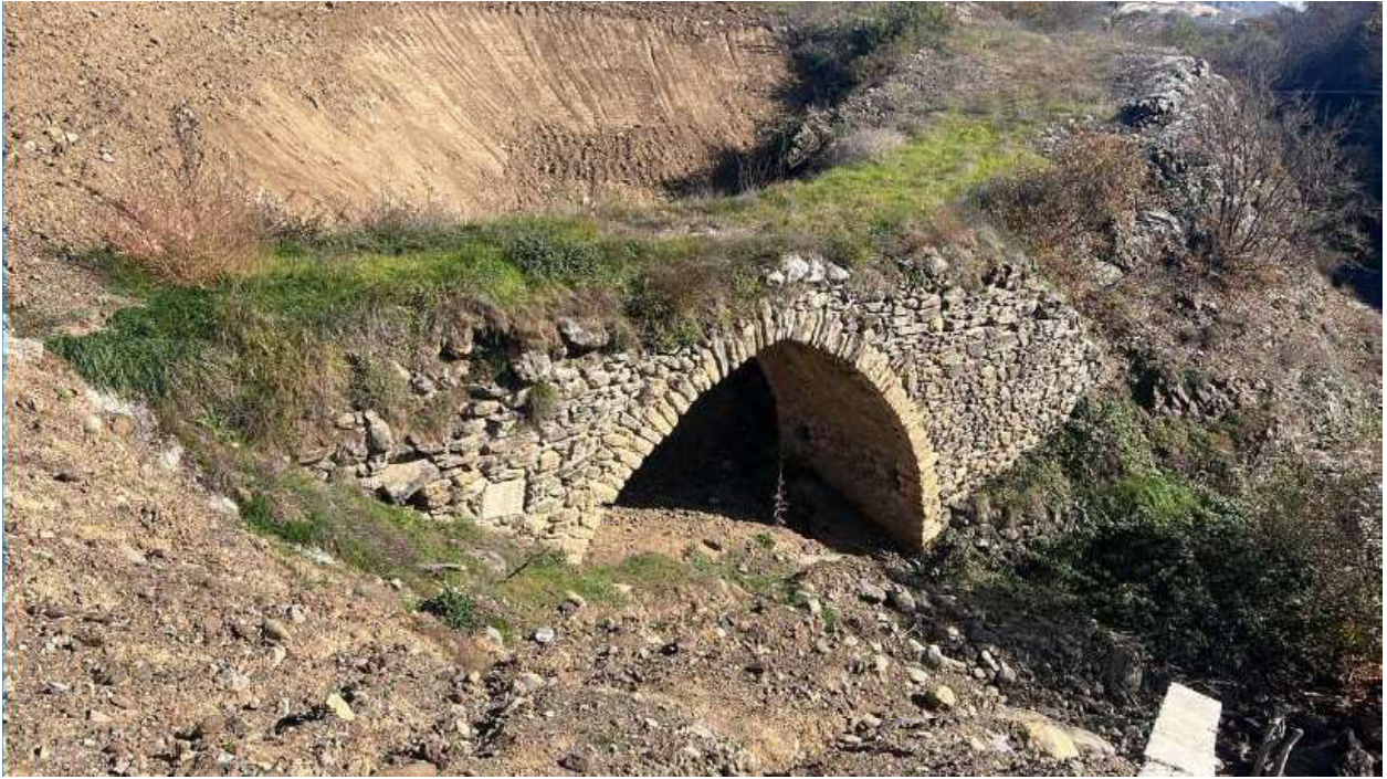
Figure 2: Photograph of Halevor Bridge Taken on 6 November 2023
